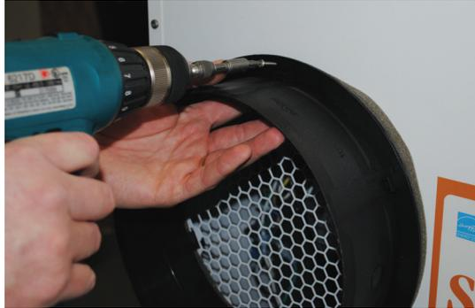
**Step 4:** If attaching duct collar to both exhaust outlets, repeat steps 2-4 for the opposite side. If only using one exhaust outlet, skip step 4 and proceed to step 5.
