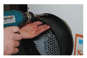
**Step 4:** If attaching duct collar to both exhaust outlets, repeat steps 2-4 for the opposite side. If only using one exhaust outlet, skip step 4 and proceed to step 5.
