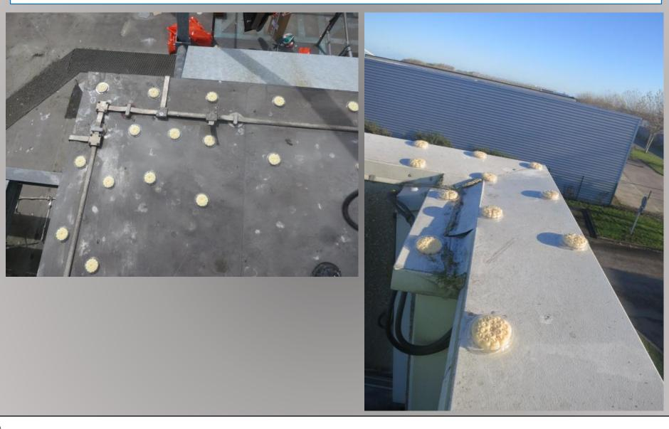
Where gulls have previously nested, or are likely to nest, dishes should be fitted to half bricks, as shown below. Where a colony of gulls has been nesting on the roof for many years, we recommend fortnightly visits during the first nesting season after treatment with optical gel, during which nests built in untreated parts of the roof should be removed and treated.
