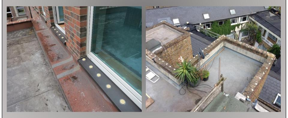
If the ledge is more than 10" deep, and there is nesting/night roosting in the immediate vicinity of the ledge, two rows of dishes should be applied. Dishes should always be fitted right into the corners of the ledge as birds favour the sheltered corners.
