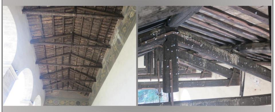
The rafters were first cleaned. Dishes of *Bird Free* were then fitted to the upper parts of the rafters at 8" centres (below left), and to the lower part of the rafters at 10" centres (below right).
