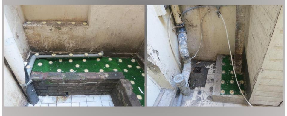
Pigeons nesting in the corner of balconies is a common problem. In this case, the nest must be removed and four dishes fixed in a square at 6" centres where the nest was.
