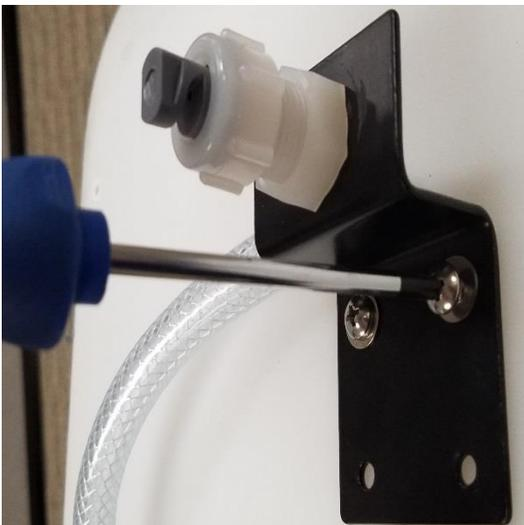
Attach Nozzle Bracket to Tank with (2) 10-24 x ¼” screws.
