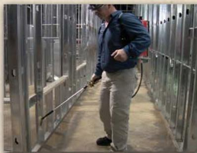
**Bora-Care Commercial is used for commercial structure new construction termite treatments.**
