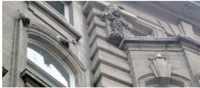
*The large number of gulls present during the summer months (more than 30 gull nests were observed on the lintels, cornices and other architectural features) was resulting in extensive fouling of the façade and the pavement below.*
