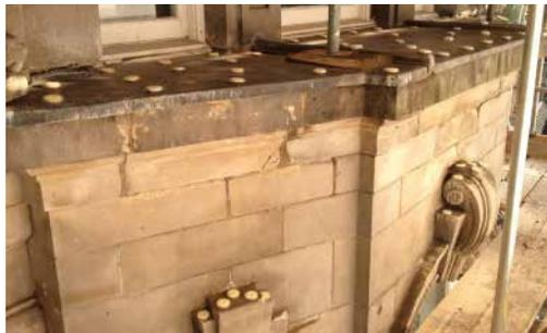
The entire façade was pressure-washed and all nests were removed. To prevent day roosting, the cornice above the fourth floor was treated with two rows of dishes of Optical Gel at 12 in. centers (left); while the deep ledges in front of the three bay windows on either side of the façade at the fourth floor were treated with three rows of dishes at 12 in. centers.
