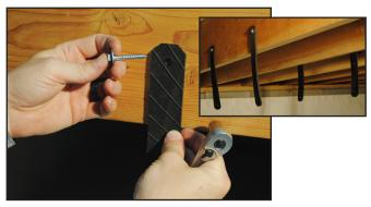
**Step 4:** Install the brackets using the J bolts to hook into the straps.
