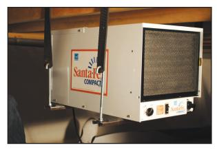
**Step 7:** Position unit into place and add the (4) Hex Head screws and the (4) 5/16" washers to secure the unit to the hang kit.
