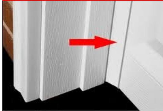
**Install Rodent Shield on the inside of the weather strip as shown below.**
