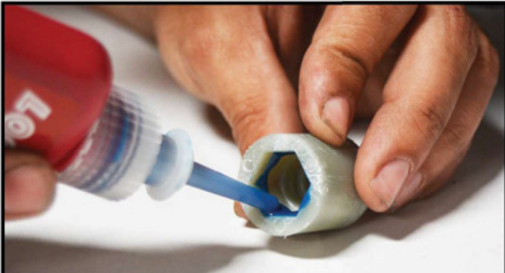
21 Use a sealant around the inside of the plastic coupling for a tight fit
